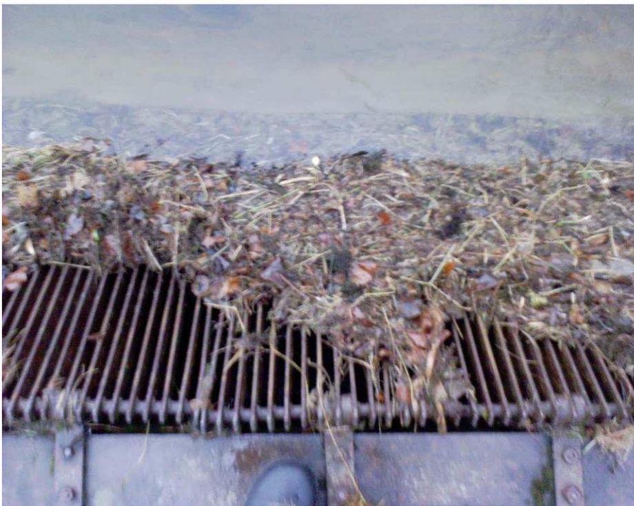
**Screen with 12mm spacing, showing restriction to flow caused by debris**
